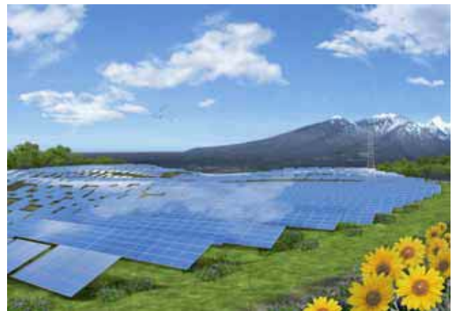
Fig. 12: Mega-watt photovoltaic system.
